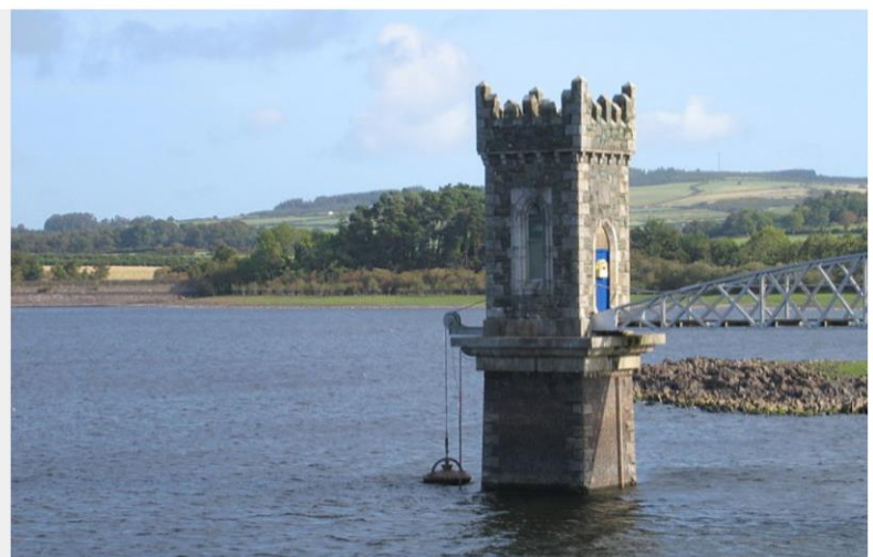
Part of the Vartry Water System
